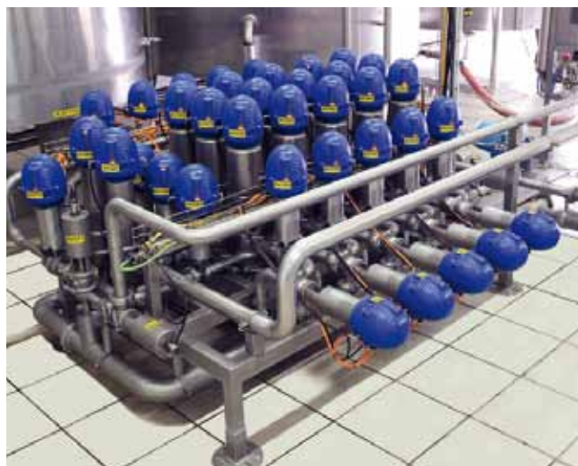
Moloko Dairy cream valve cluster with Alfa Laval Unique SSV, Unique Mixproof and LKB valves and ThinkTop valve sensing and control units.
