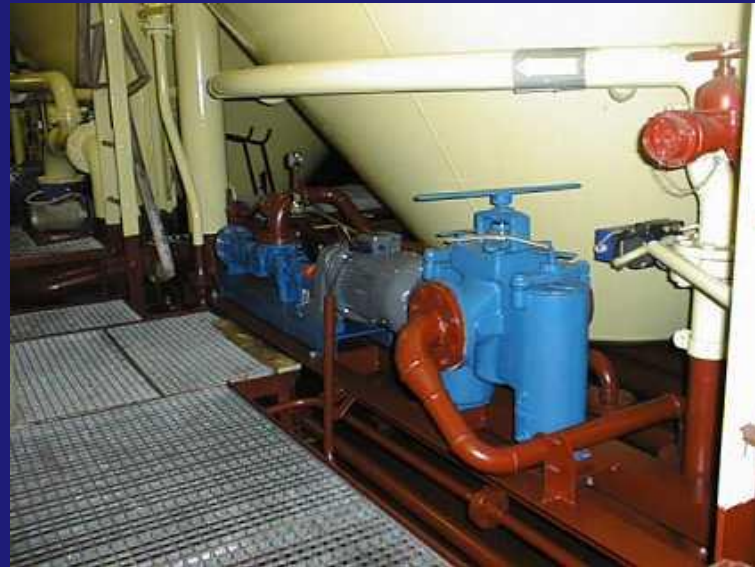
Duplex strainer. (Taking out particals above 3-4mm)
